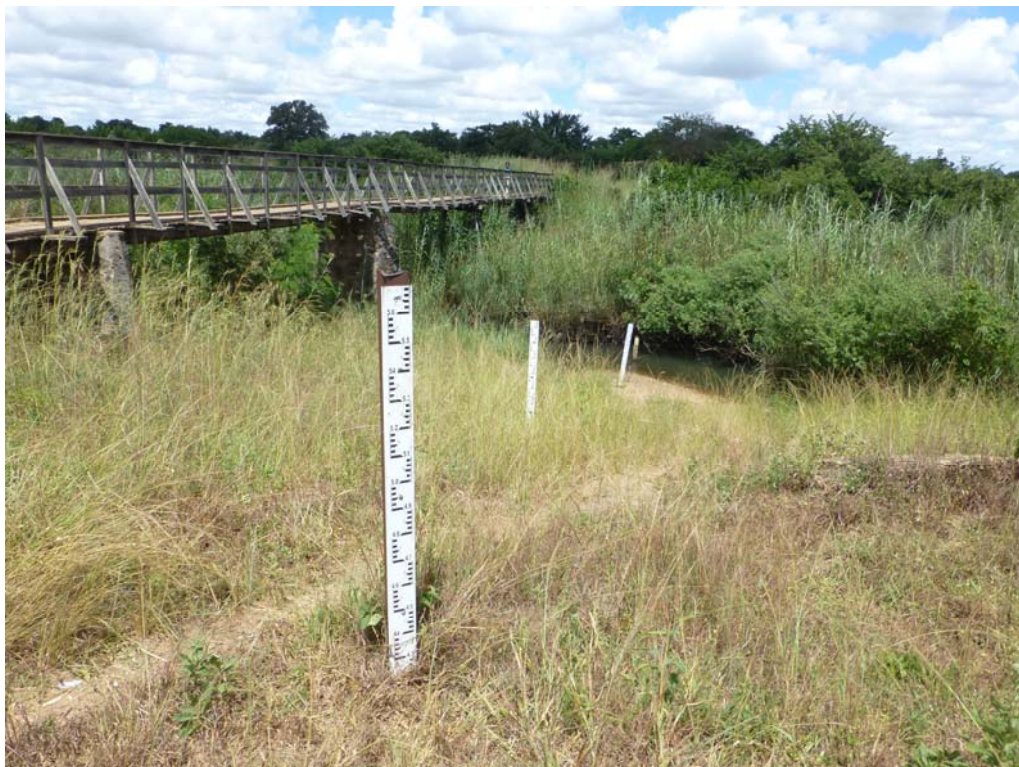
Figure 6: Gauging station 5-024 on Chongwe river after Ngwerere confluence, March 2015.
