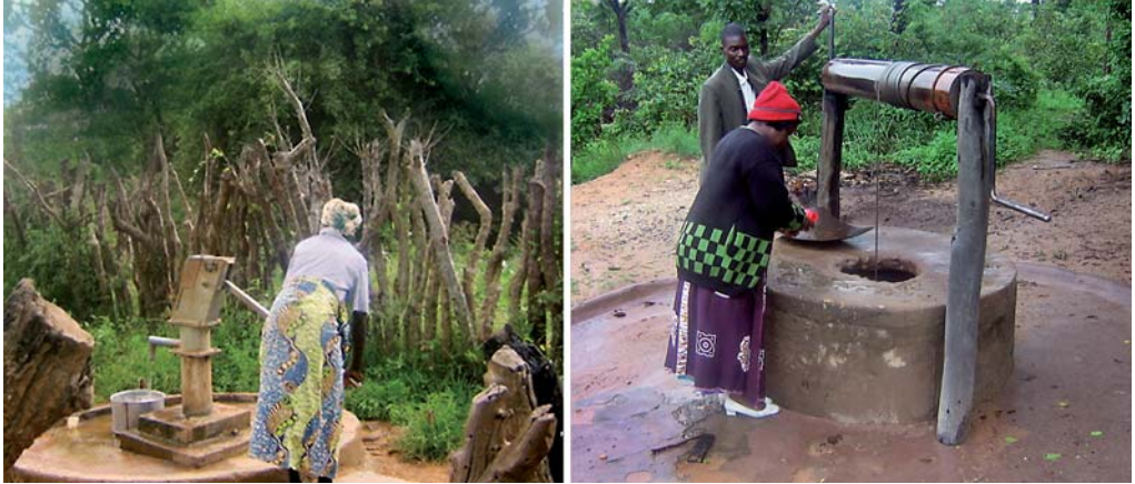
Figure 18: The two most common water point types: Handpump of type India Mark II (left) and hand dug well with bucket and windlass (right).
