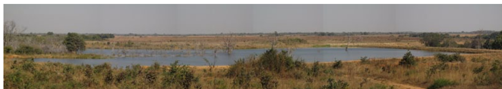
Chunga earth dam
