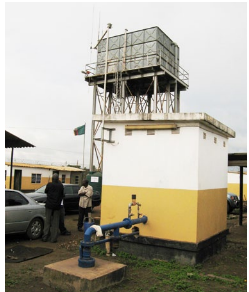
Local water supply from borehole, Kanyama, Lusaka City
