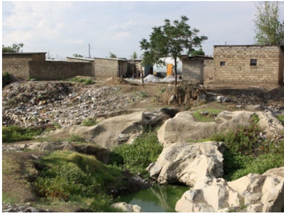
Unprotected area on the Lusaka Dolomite with pit latrines, garbage disposal and quarrying around an open groundwater surface.
