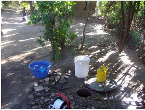
Unsafe forms of water supply: unprotected shallow well and open groundwater surface used as dumpsite and for water supply
