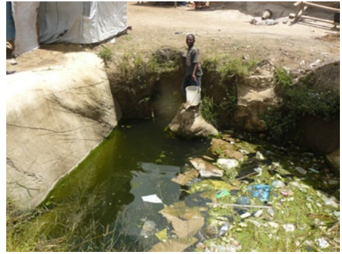
Unsafe forms of water supply: unprotected shallow well and open groundwater surface used as dumpsite and for water supply
