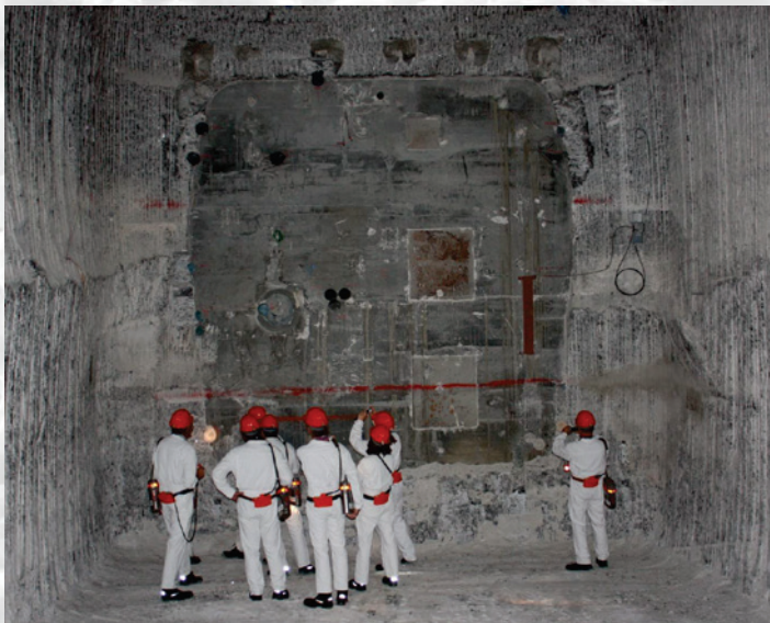
dimension of the construction: height: 3.7 m to 5.0 m, width: 4.6 m, length: 25 m (this real full scale experiment represent a typical drift seal profile.)
